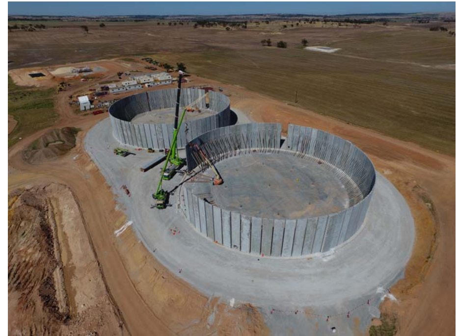
Construction of the Cunderdin storage tanks
