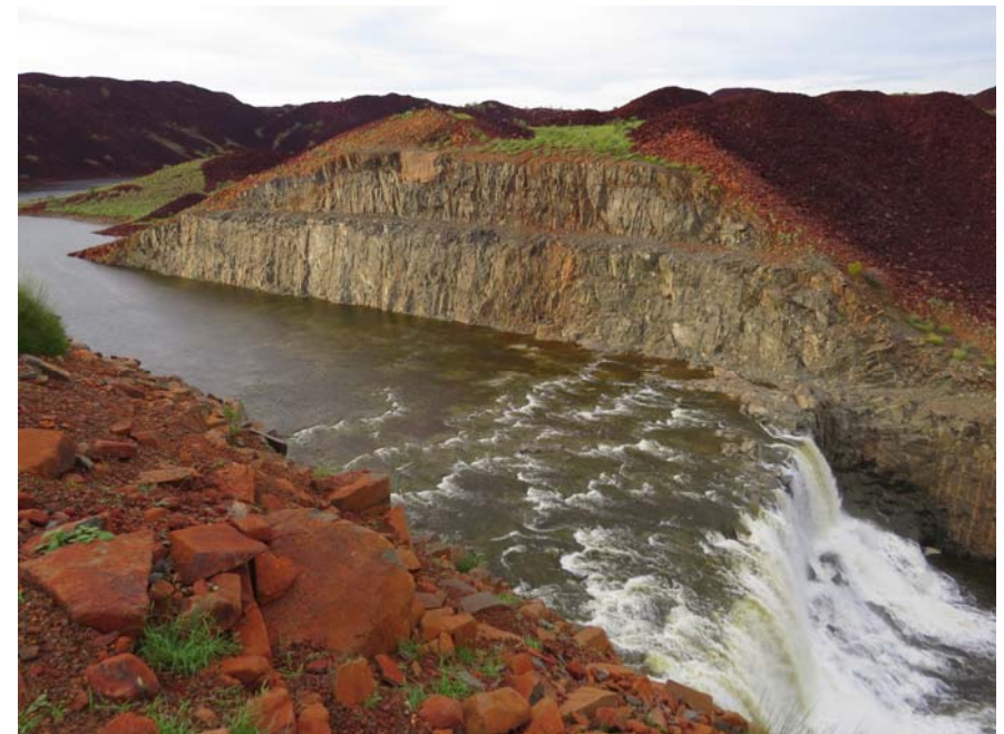
Harding Dam Overflowing
