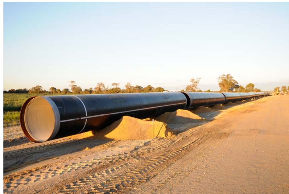
Harvey pipeline construction
