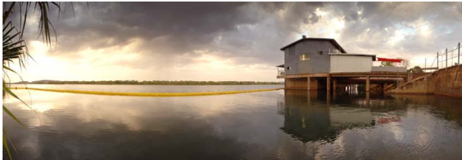
Kununurra Pump station
