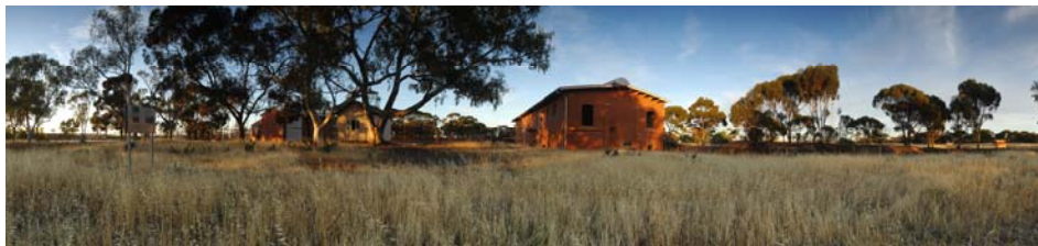
Merredin Pump Station
