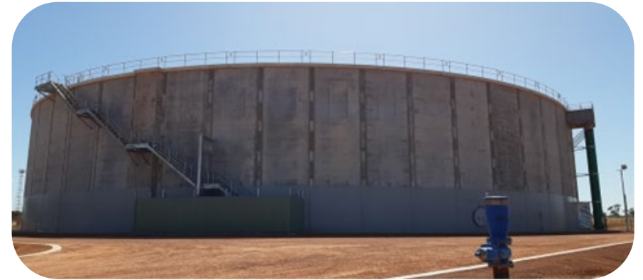
Figure 23: New sealed water tank in Merredin
