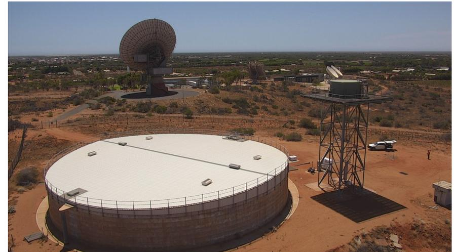
**Figure 1: Carnarvon ground level and elevated tanks**
