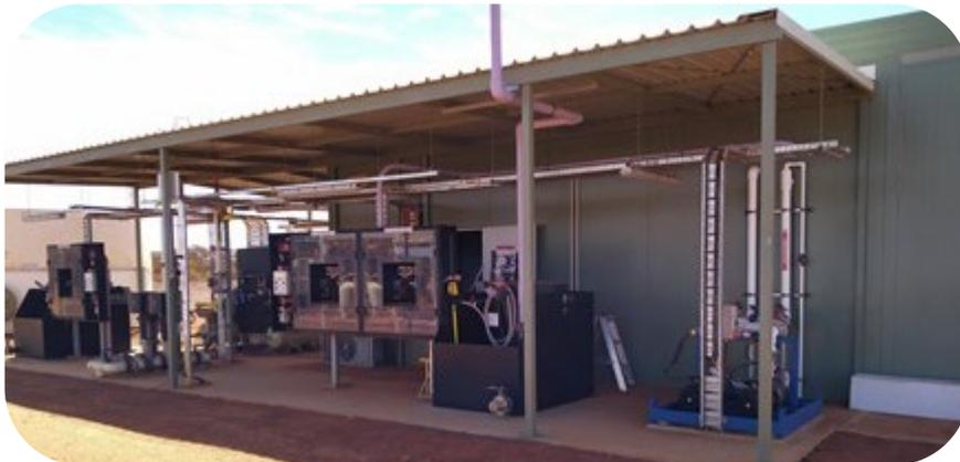
Figure 16: Mt Magnet EDR plant – feed pump and chemical dosing
