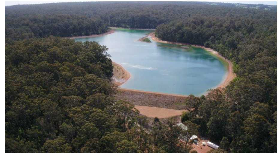
Figure 3: Manjimup (Scabby Gully) Dam
