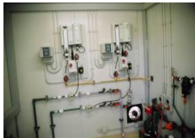
Disinfection (chlorination)
