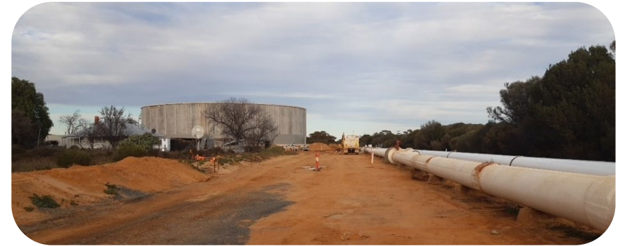
Figure 26: New sealed water tank in Dedari
