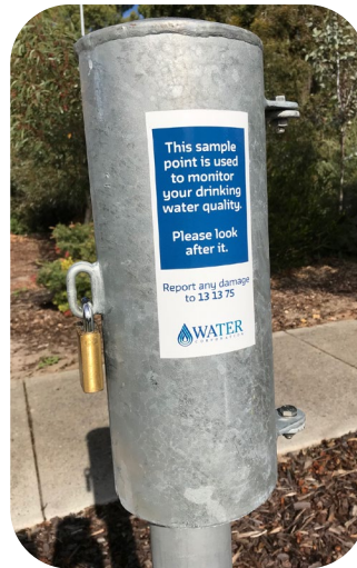
Figure 20: Suburban water sampling point
