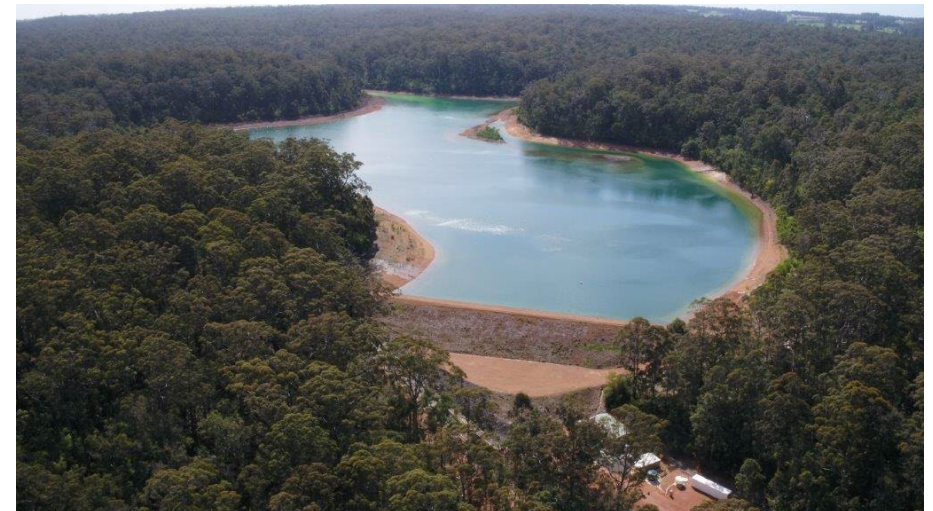
Figure 3: Manjimup (Scabby Gully) Dam
