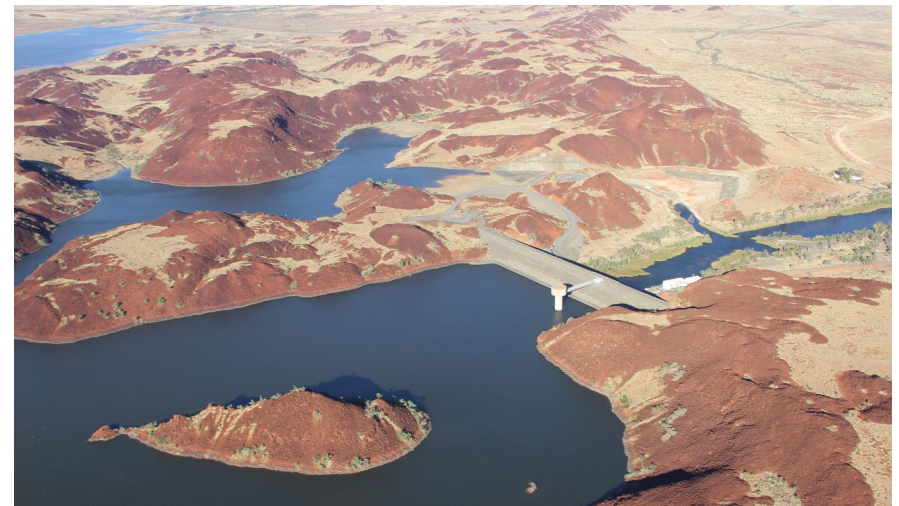
Figure 14: Aerial view of Harding dam (North West Region)
