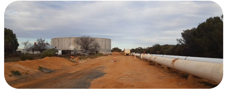
Figure 26: New sealed water tank in Dedari
