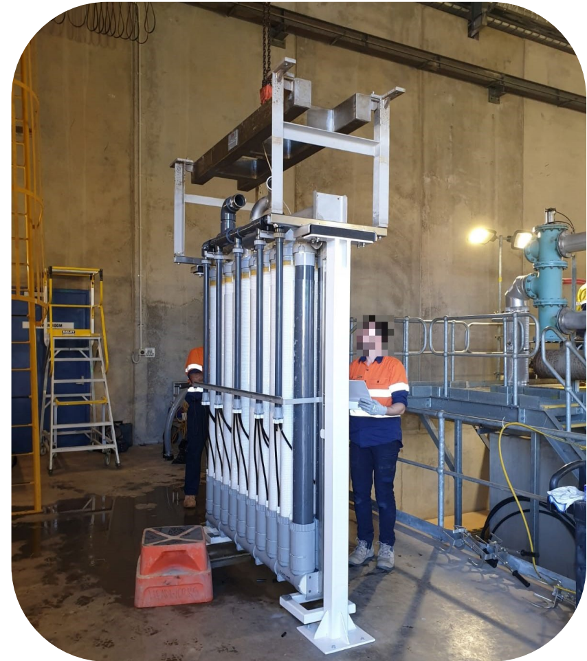
Figure 27: Harding membrane train
