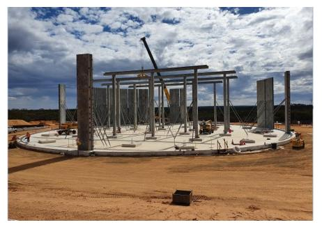
Figure 37: Sealed water tank construction in Dedari
