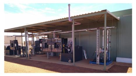
Figure 27: Mt Magnet EDR plant - feed pumps and chemical dosing systems
