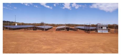
Figure 28: Mt Magnet 200-Kilowatt solar panel system - the entire site is powered from solar power
