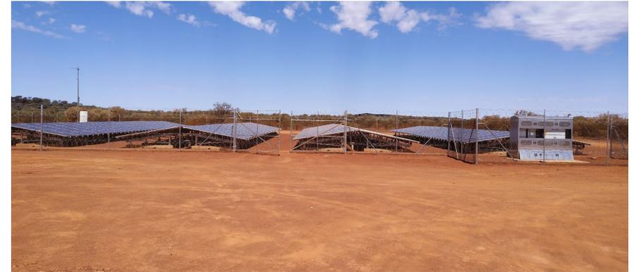
**Figure 28: Mt Magnet 200-Kilowatt solar panel system - the entire site is powered from solar power**
